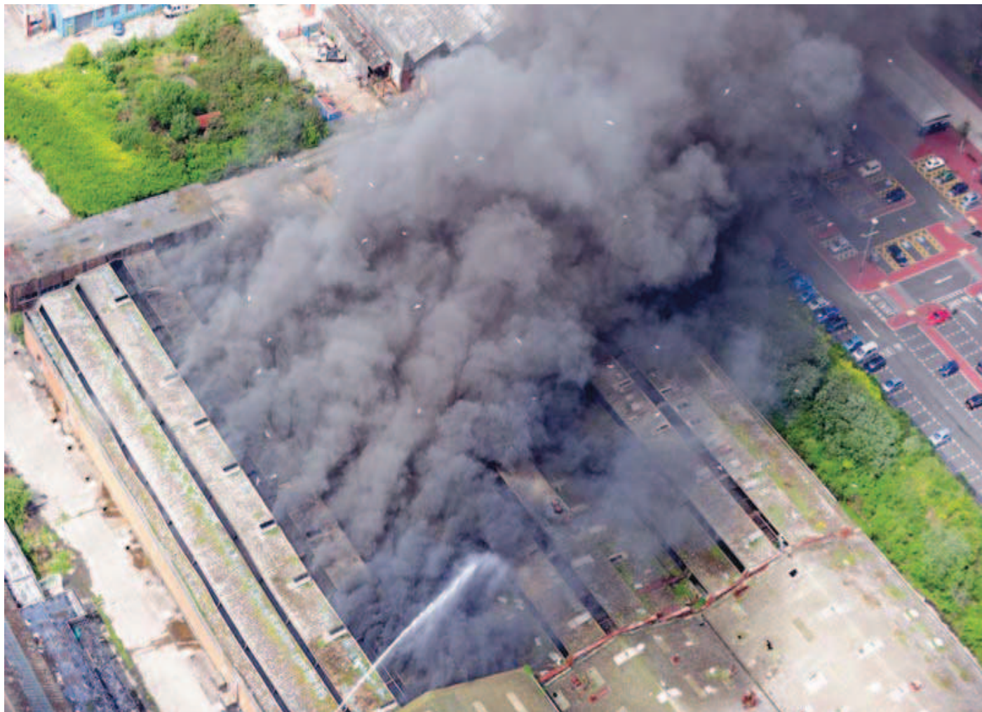
Photograph 2 – Fire at a depot in Swansea in June 2011 where tyre wastes were stored led to a major incident that lasted several weeks, threatened the evacuation of thousands of nearby residents, and cost the local authority and emergency services about £1.5 million.
